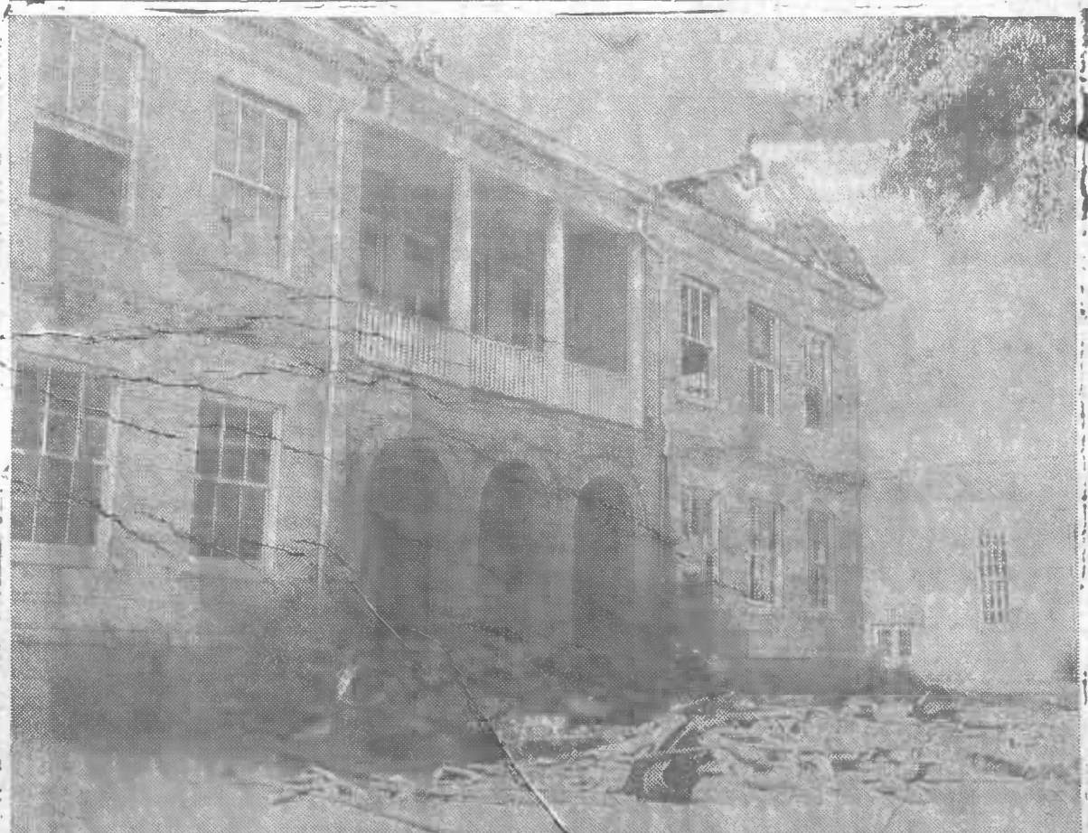
RAZING BEGINS ON OLD IUKA SCHOOL—Demolition crews are making rapid progress reducing this old school building to stacks of bricks, timbers and piles of rubble as one of Iuka's old landmarks gives way to progress. The building was constructed in 1909 and first opened to classes in 1910 as the Iuka Female College. Some years later it became the Iuka Normal Institute and lately has been the Iuka Municipal Separate School. Students who attended classes here last year will be housed in a brand new building just to the rear of this one. The basement will be filled in and the ground leveled where the building now stands, possibly to be used as a playground. Jack McKelvy, Florence, Ala., has the wrecking contract.
